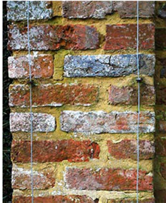
Tricks of the trade: many wires hold climbing plants in place.
